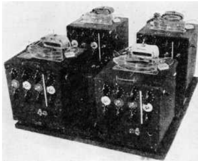
Figure 5.2: Ashby's electro-mechanical homeostat.
